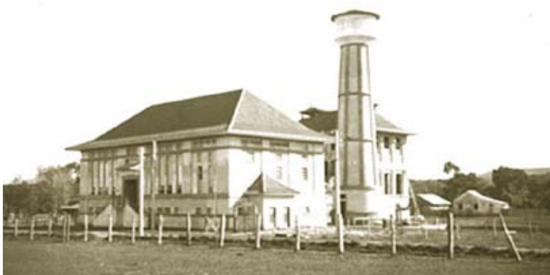
Antiga Usina Municipal
