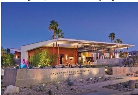
Figura 40- Fachada Palm Springs
